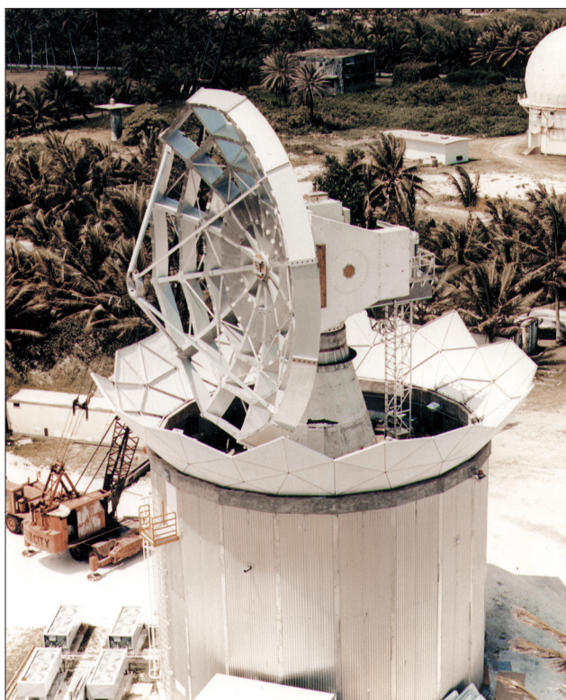
FIGURE 10. The radome surrounding the MMW radar is being erected around the radar during construction. The right image shows the radar as it appears today surrounded by its radome.
