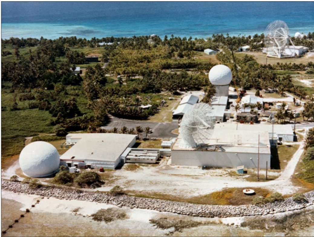
FIGURE 2. The island of Roi-Namur at the northern extreme of the Kwajalein Atoll is the location of the four primary KREMS radars. Looking southwest from the ocean side reef, ALCOR is seen in the lower left corner, TRADEX in the center foreground, MMW in the center background, and ALTAIR in the upper right corner.
